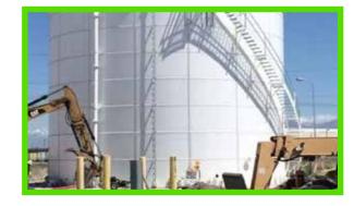
**Efficiency**- Fewer pieces to fabricate mean fewer pieces to unload and install. Our powder-coated epoxy panels are 116" x 58" coverage sidewall sheets. Other companies use smaller, non-standard coverage sheets. This leads to a 10% to 22% increase in sheets to cover the same capacity as our tank construction. We save you time and money.
