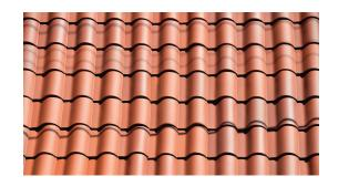
**Terracotta** - In warmer climates, algae and moss will also grow on terracotta roofs. However, this will be a lot slower than concrete. This type of roof is suitable as long as it is kept clean. Cleaning is often done by spraying the roof down with chlorine.
