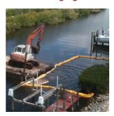
Turbidity Curtain, Dewatering Tubes, and Secondary Containment
