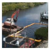
Turbidity Curtain, Dewatering Tubes, and Secondary Containment
