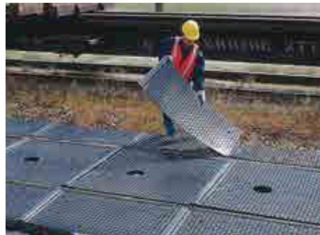
Track Pans with Grates and Covers
