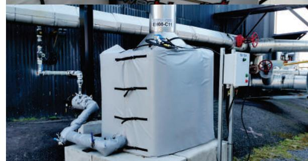
Powerblanket supplied the custom frac tank heating system currently working on-site. The heating system installed quickly despite rainy weather, and has protected the contents from freezing.
