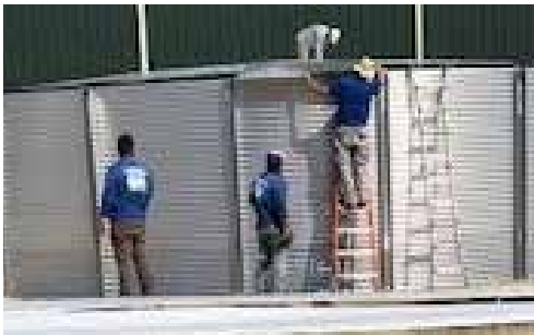
Figure 17 Putting on 535" Roof Sheet (1st Sheet)
