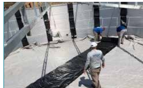
Figure 13 Liner Rolled out perpendicular to bulkheads
