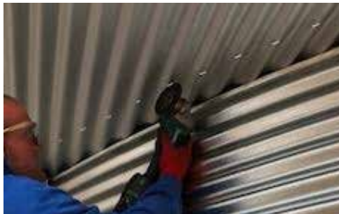
Figure 18 Using Grinder to mark the Roof
