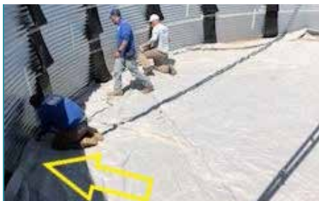
Figure 12 Rolling the Geotextile Up on the Tank Wall
