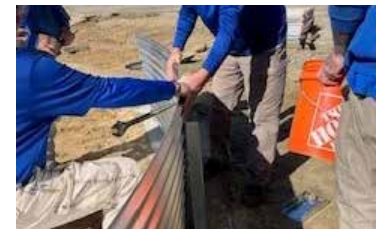
Figure 5 Forming the First Ring of Tank
